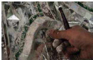
Pic 8. Mirror Pieces Installation (Same)
